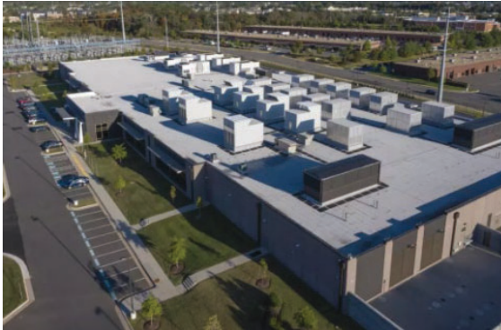
Facebook leased data center (Ashburn, VA) 70+ MW (~50,000 homes)
